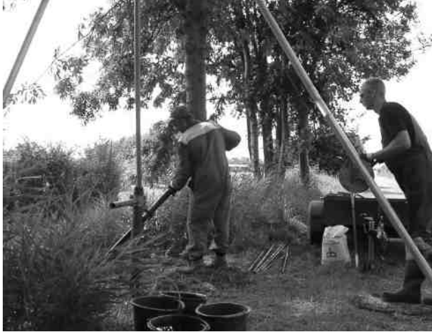
Figure III-2.2-ii.9a Example of hand pulsing, using tripod and steel casing
