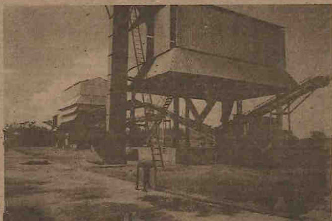
The municipal solid waste composting plant at Tiruppur.
