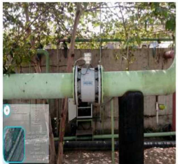
M/s.Chemplast Sanmar Limited Plant –I
