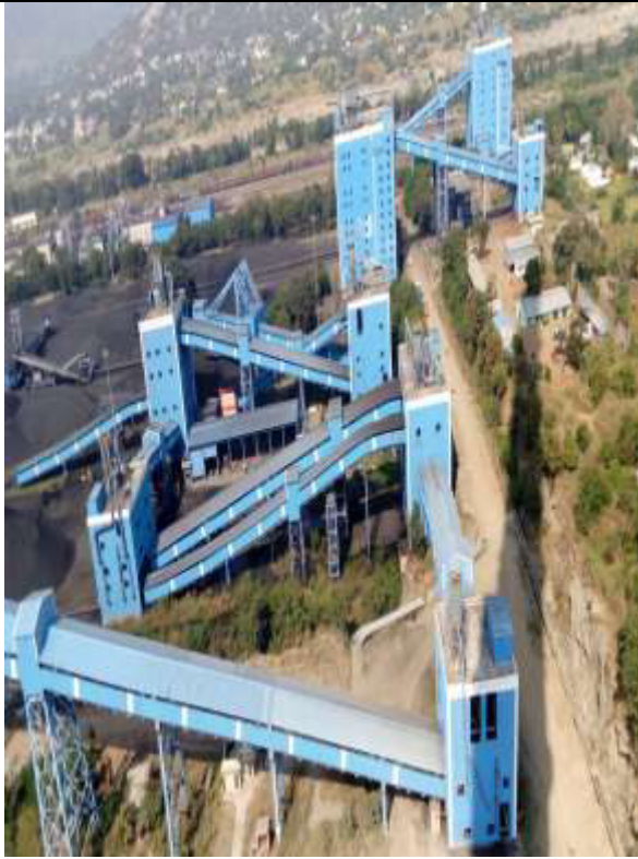
Coal yard covered with sheets-MTPS II
