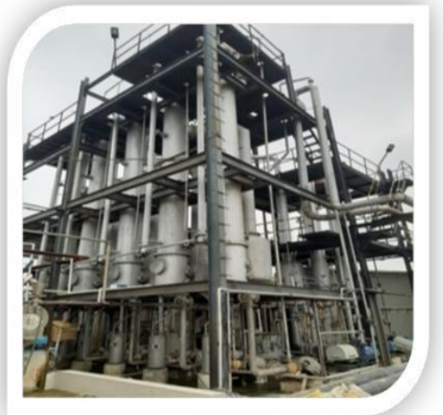
Multiple Effect Evaporator – Falling Film
