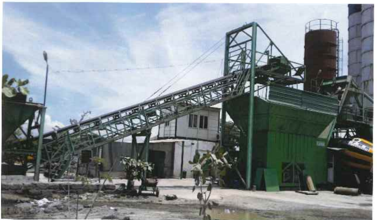
Conveyors without covering
