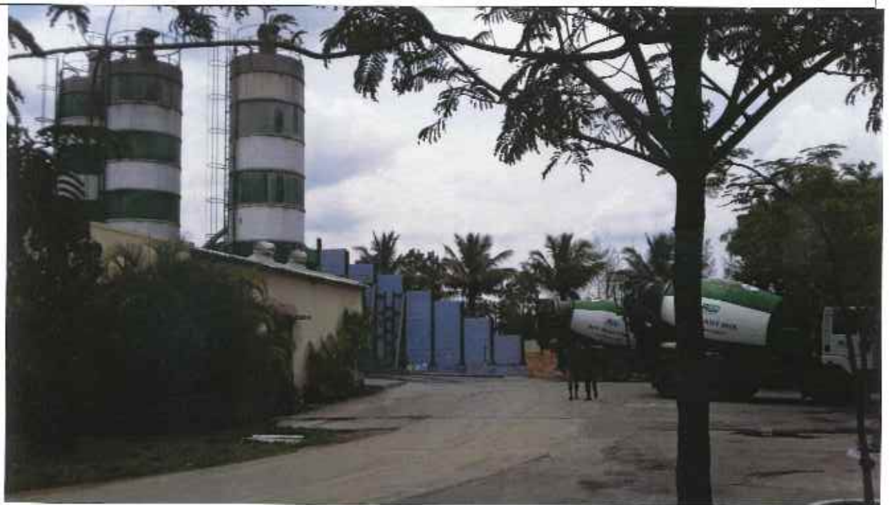
Paved Roads within RMC Plant
