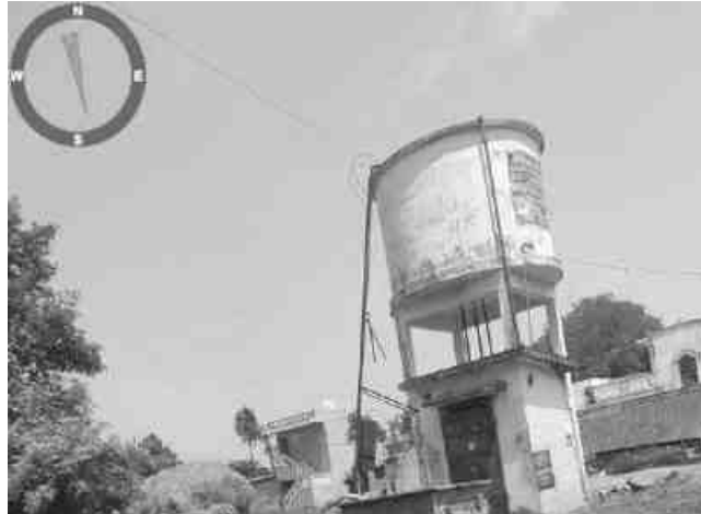
Menallur – Overhead Water tank
