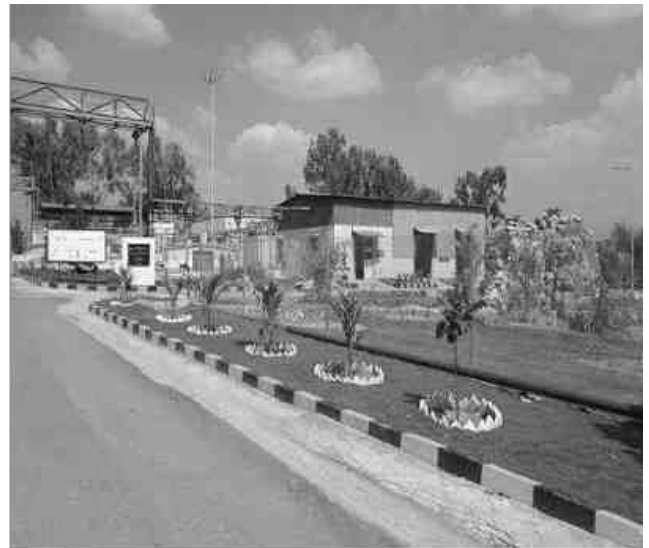
ETP and STP
