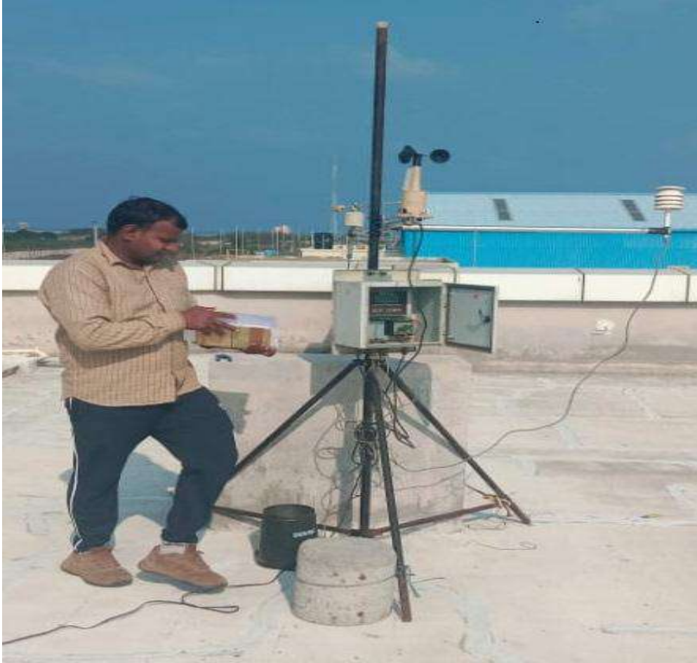
Figure 3.2: Meteorological Station Installed at Project Site
