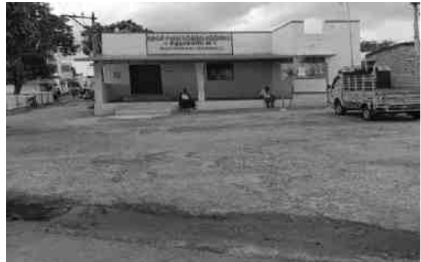
Community Hall, Ramalingapuram
