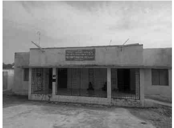
Village Service Centre, Ponakudi
