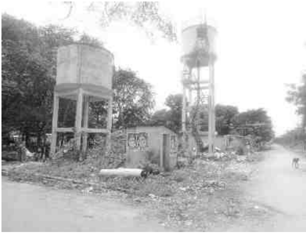
Water Tank, Samnathapuram
