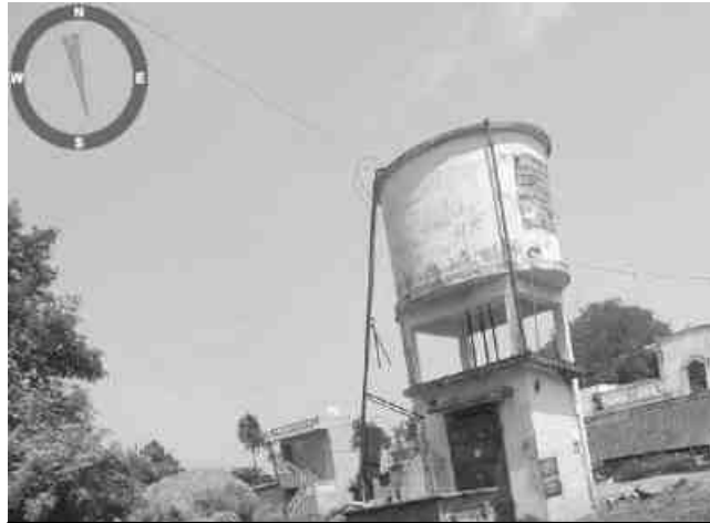
Menallur – Overhead Water tank
