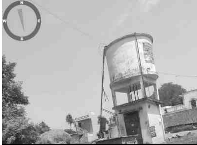
Menallur – Overhead Water tank
