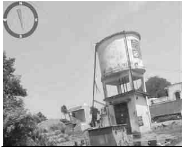
Menallur – Overhead Water tank
