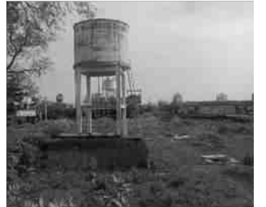
Water Tank, Alagulam
