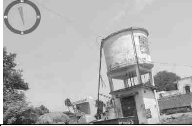
Menallur – Overhead Water tank
