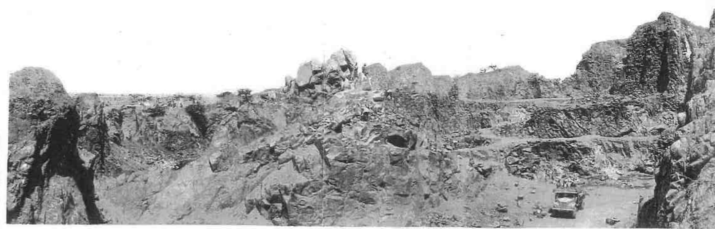
Plate 2 : Transportation of Quarried Material to Crushers.
