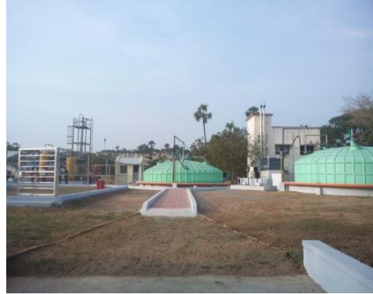
Bio-CNG Plant- 10 MTD, MWC, Chennai
