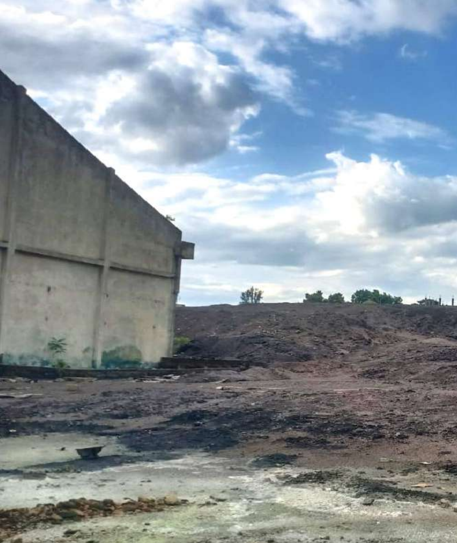
Image showing contamination of Tamil Nadu Chromates and Chemicals Ltd., premises with chromium bearing hazardous waste.
