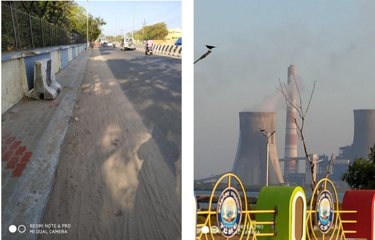
Figure 10 Roadside Suspended Dust Particles and Power Plant of Thoothukudi
