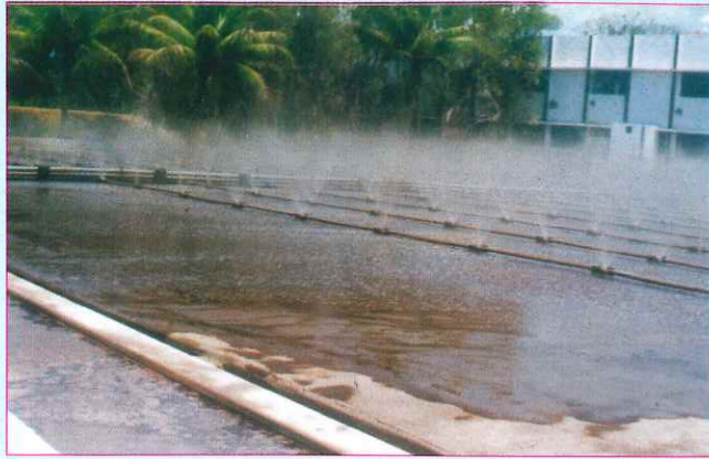
IMPROVISED SOLAR EVAPORATION PANS PROVIDED IN ONE OF THE ZERO DISCHARGE UNITS.
