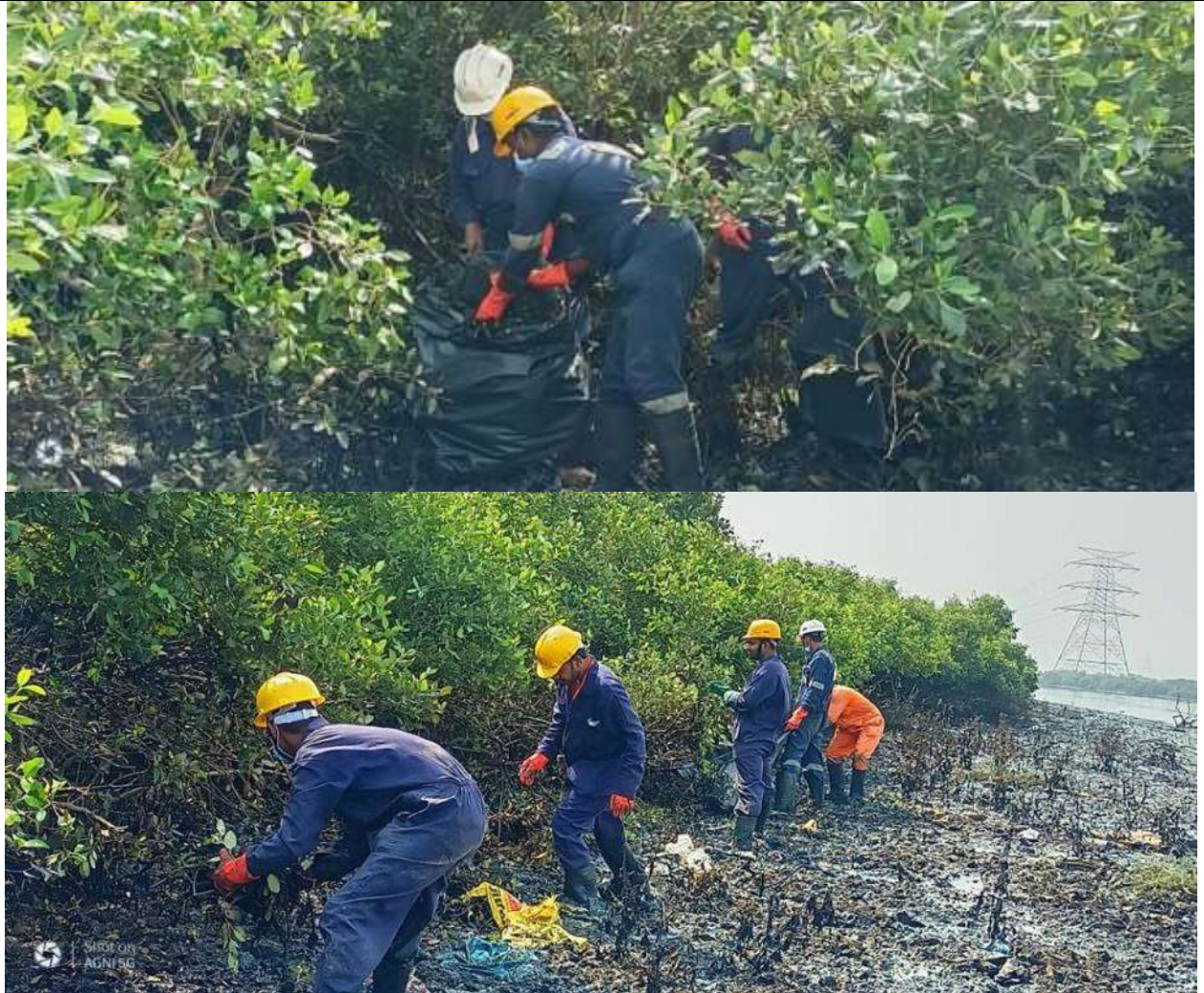
Removal of oily water out through Gully suckers at CMDA Steel yard area
