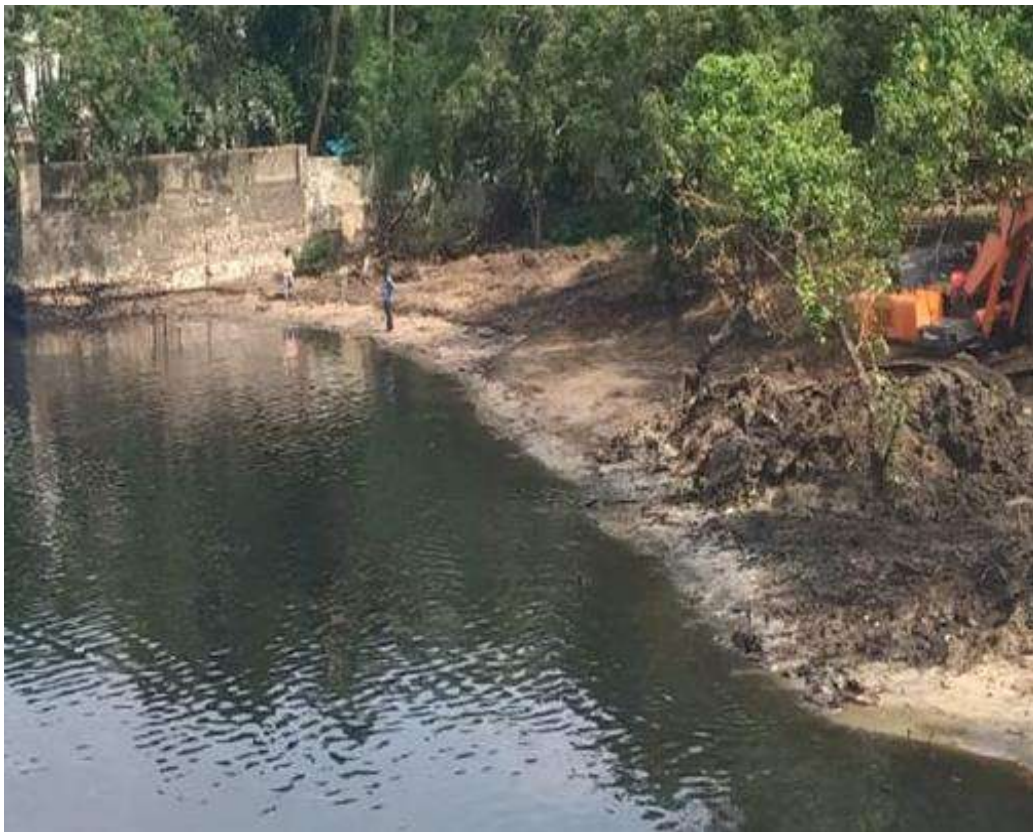
Ennore Bridge - Right Side after Cleaning
