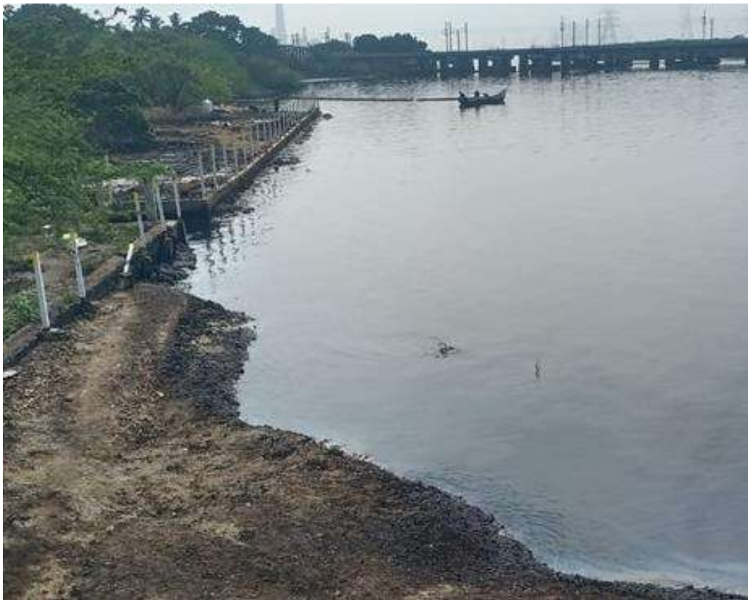
Ennore Bridge - Left Side after Cleaning
