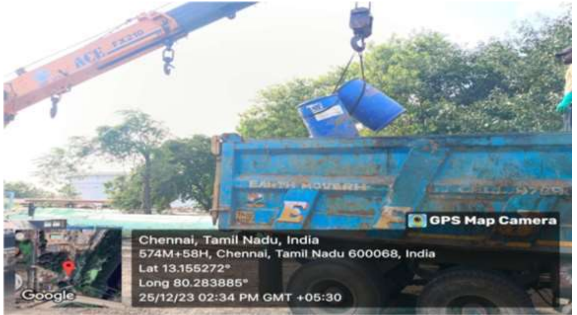
Cleaning activities in progress at Nettu Kuppam and Ennore Kuppam area
