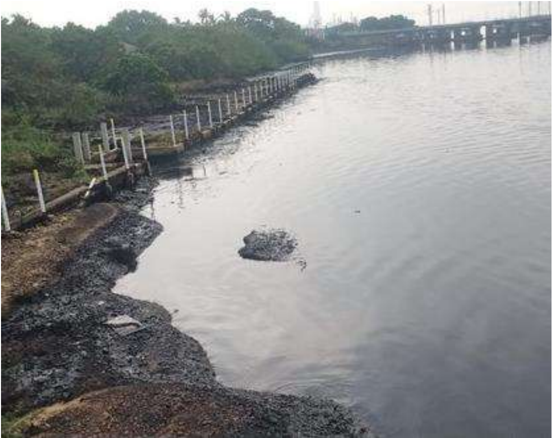
Ennore Bridge - Left Side before Cleaning
