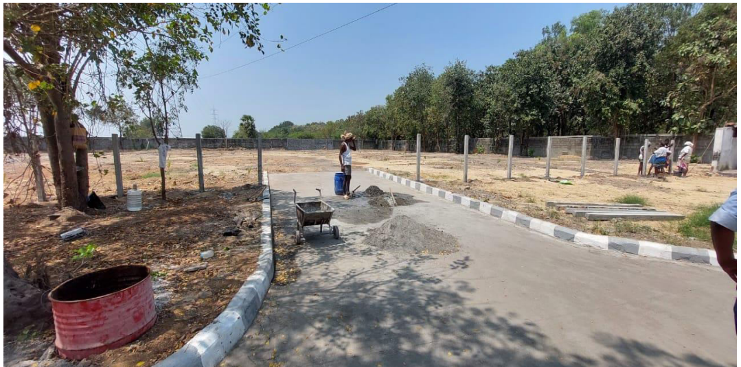
Vacant area in western direction,( where green belt can be developed )
