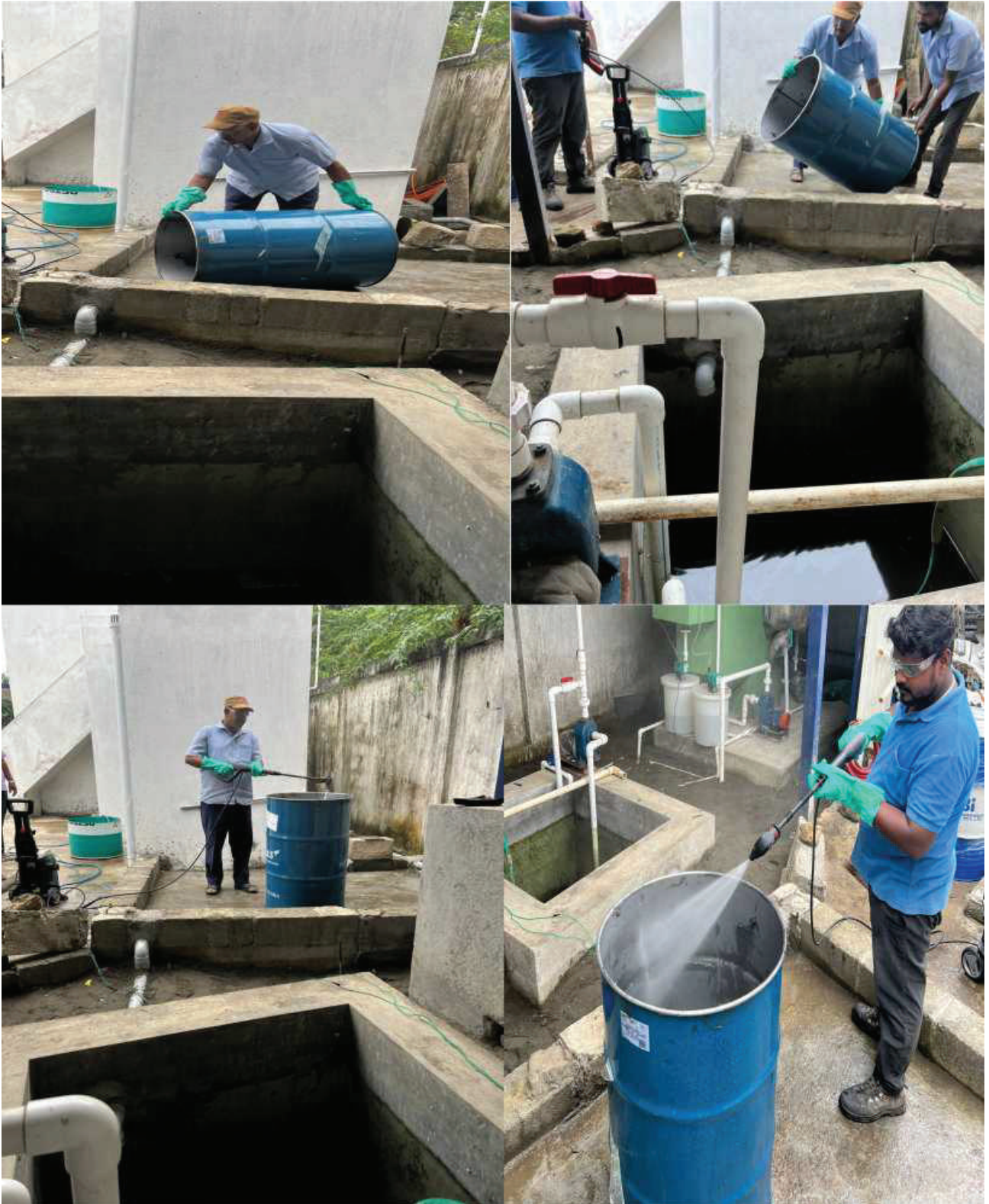
Cleaning & Emptying of Contaminated Drums on site
