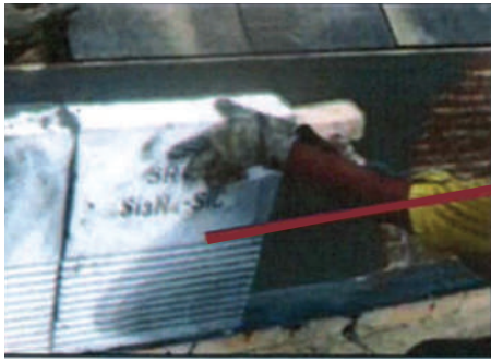
Figure 2: Fresh Silicon Carbide bricks installation in Side Wall of Pot.
