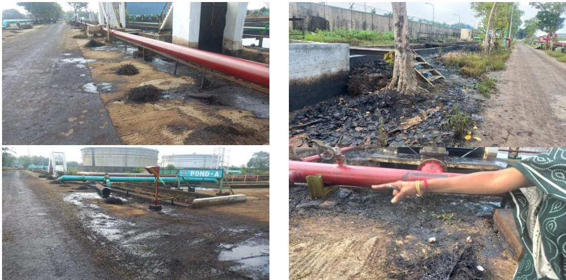
Oil spillage observed around Storm water collection Pond A
