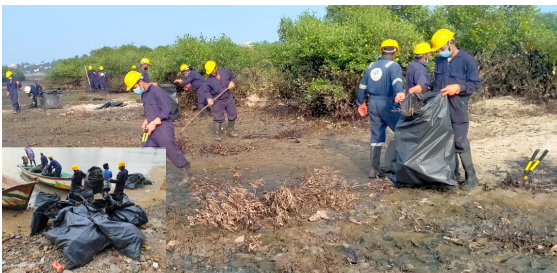
Cleaning operations at Ennore mangrove forest area by trained manpower
