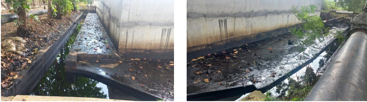
Oil Sludge storage tanks and their surrounding area
