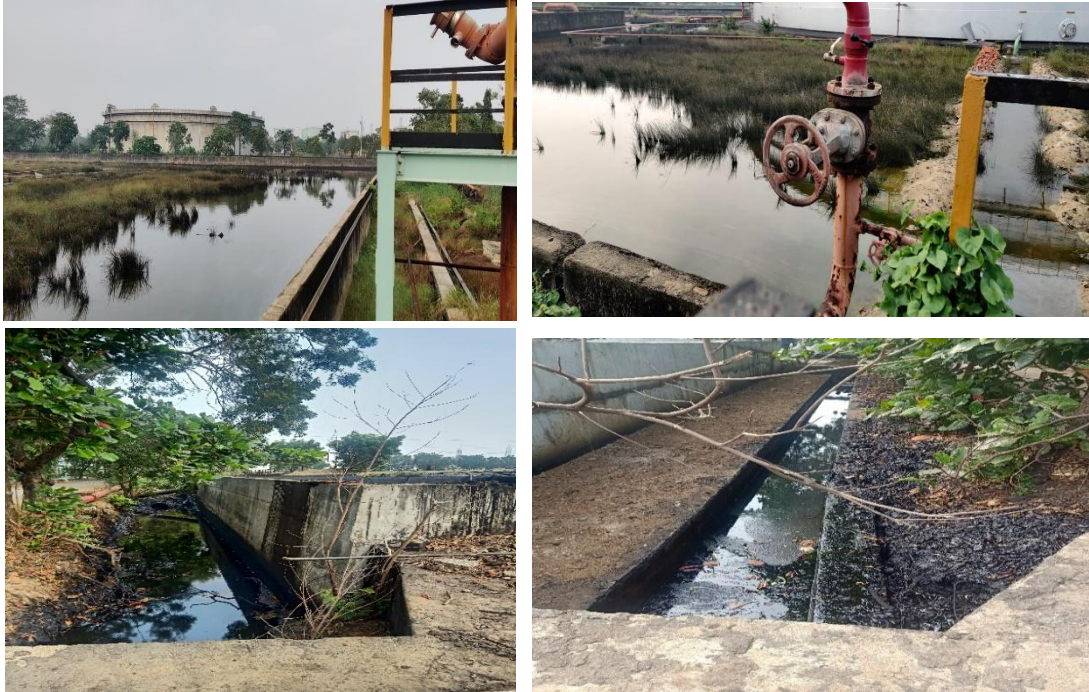
Photo showing oil spillage along drain passing adjacent to sludge storage and crude oil storage tank
