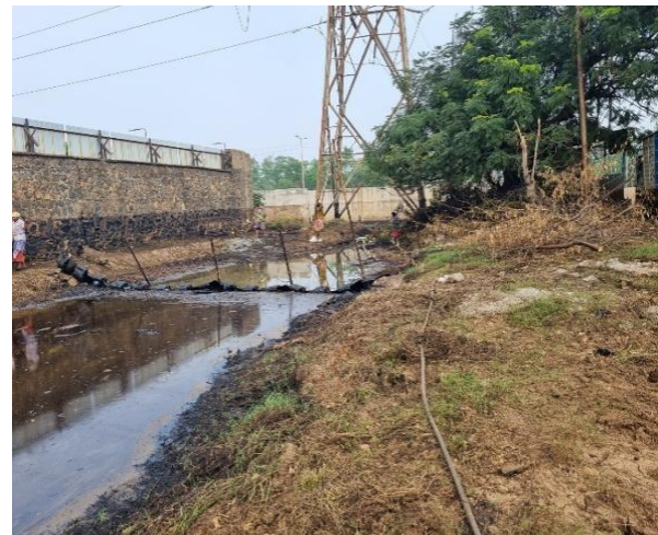
Photos showing oil / oil laden water from CPCL found its way into the storm water drain passing through the CMDA steel yard
