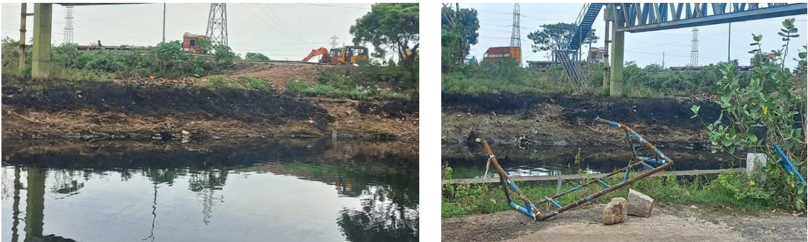
Oil Spillage observed on side walls of Buckingham canal
