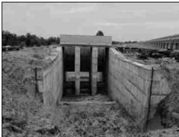
Fig No 2.8 Head sluice of south rajan channel
