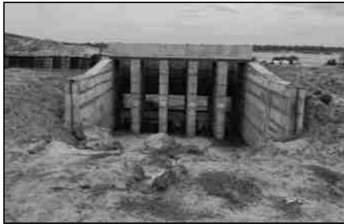
Fig No 11.1 Head sluice of north rajan channel
