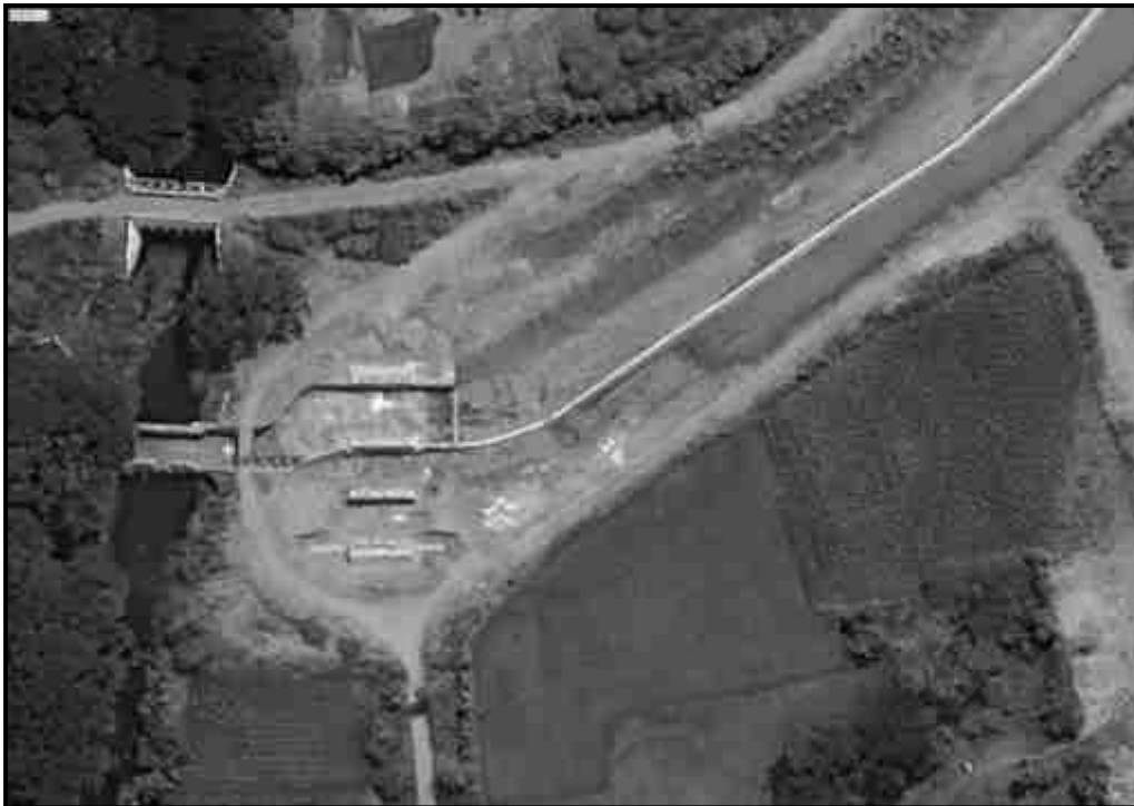
Fig No 2.9 Diversion of Narimudukku Drain into existing south rajan channel by constructing baffle wall at the centre of channel
