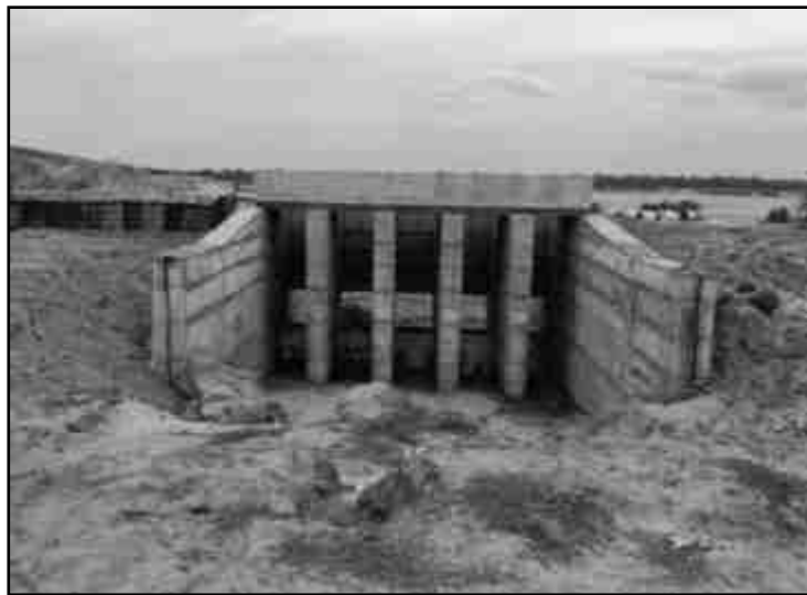
Fig No 2.7 Head sluice of north rajan channel
