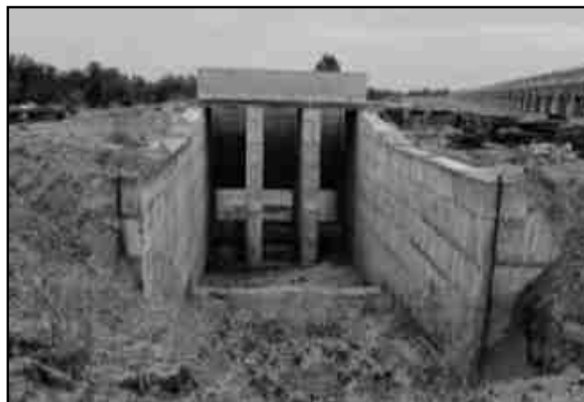
Fig No 11.2 Head sluice of south rajan channel
