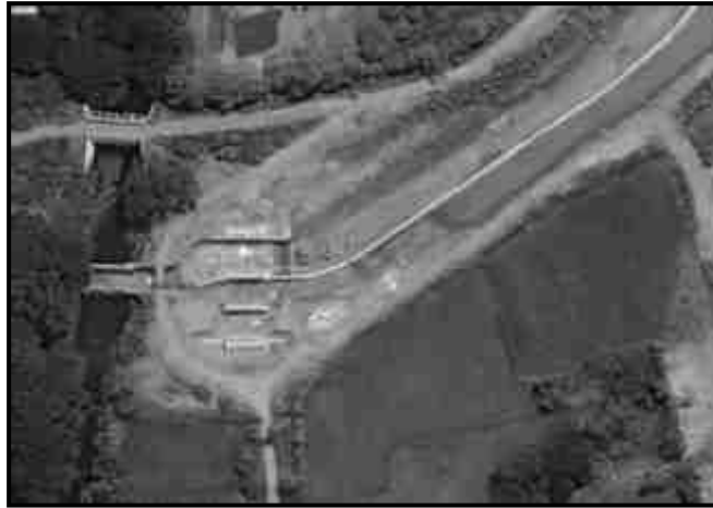
Fig No 11.3 Diversion of Narimudukku Drain into existing south rajan channel by constructing baffle wall at the centre of channel
