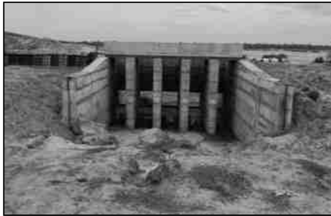
Fig No 11.1 Head sluice of north rajan channel
