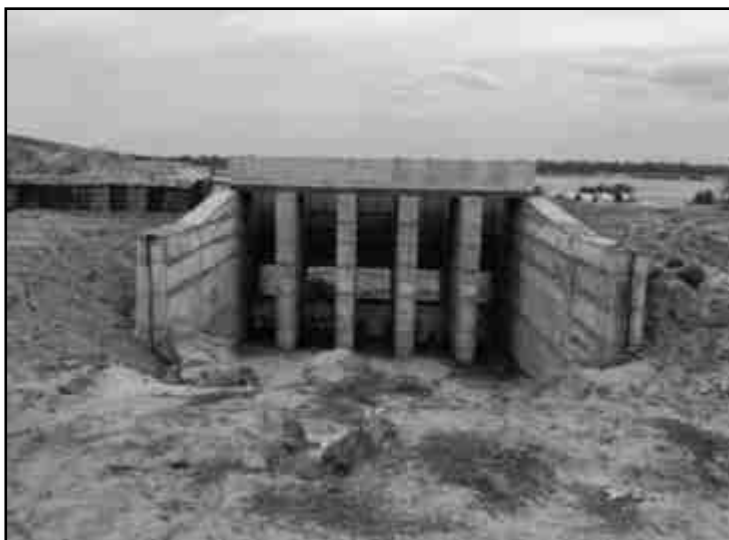
Fig No 2.7 Head sluice of north rajan channel
