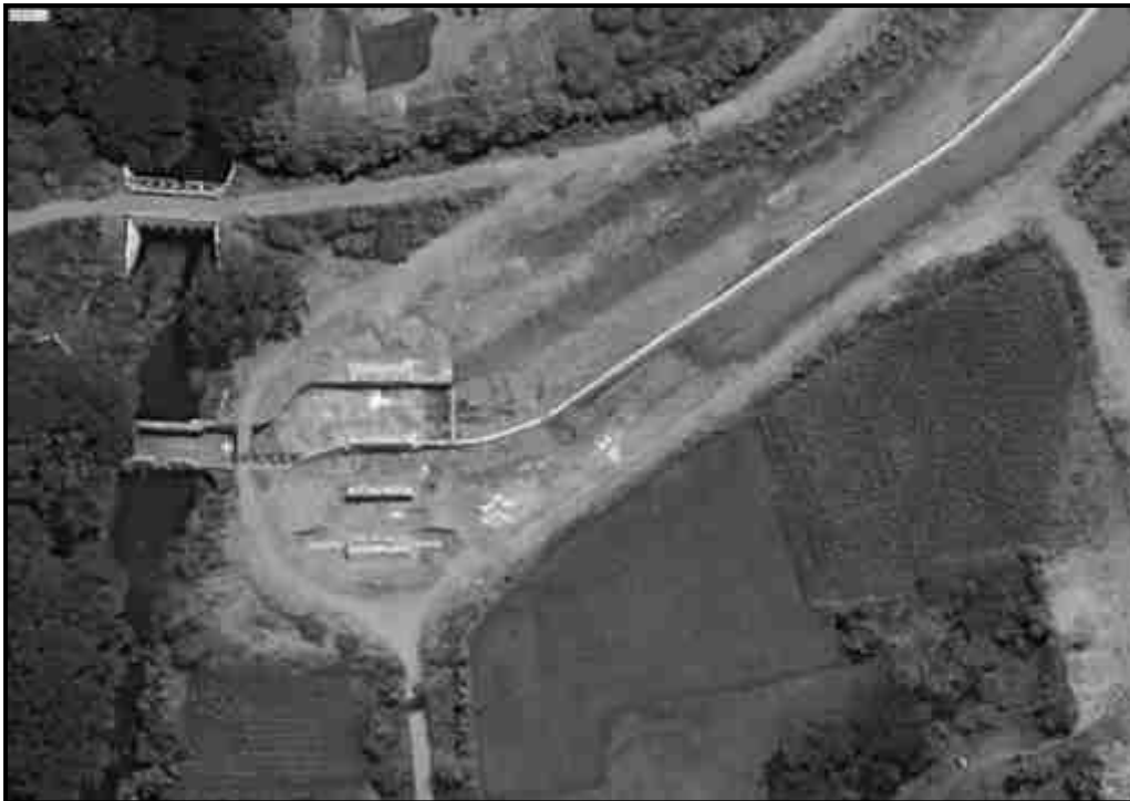
Fig No 2.9 Diversion of Narimudukku Drain into existing south rajan channel by constructing baffle wall at the centre of channel
