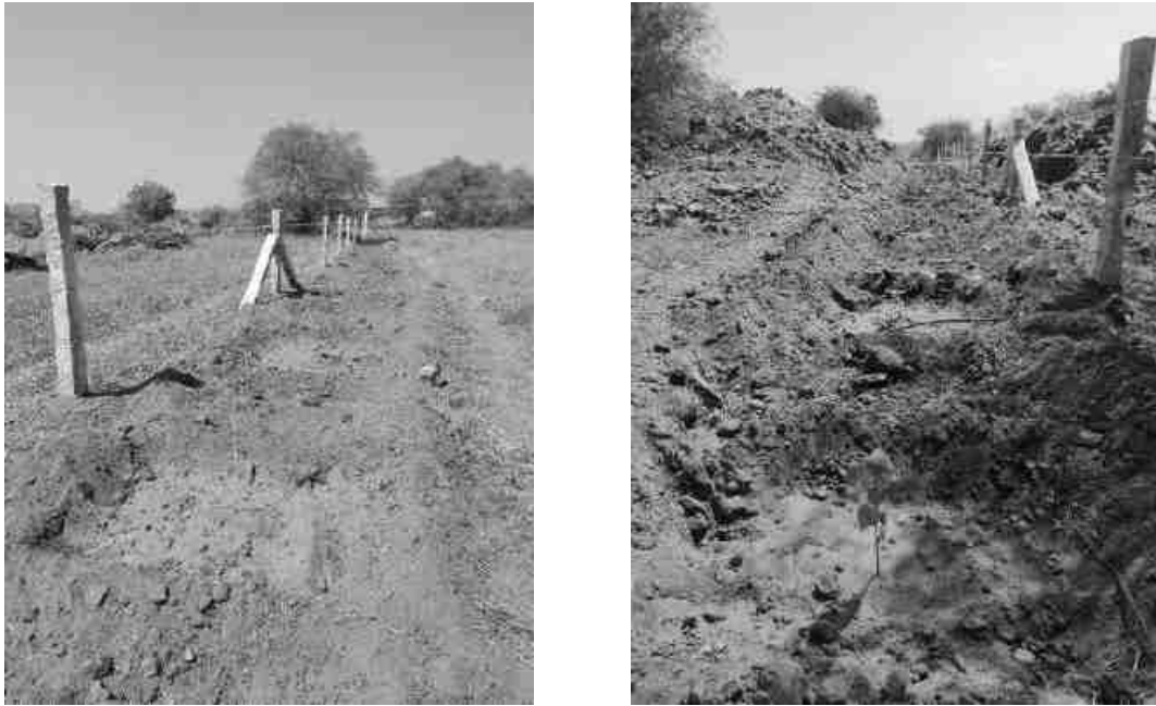
Fencing & Greenbelt at Project site
