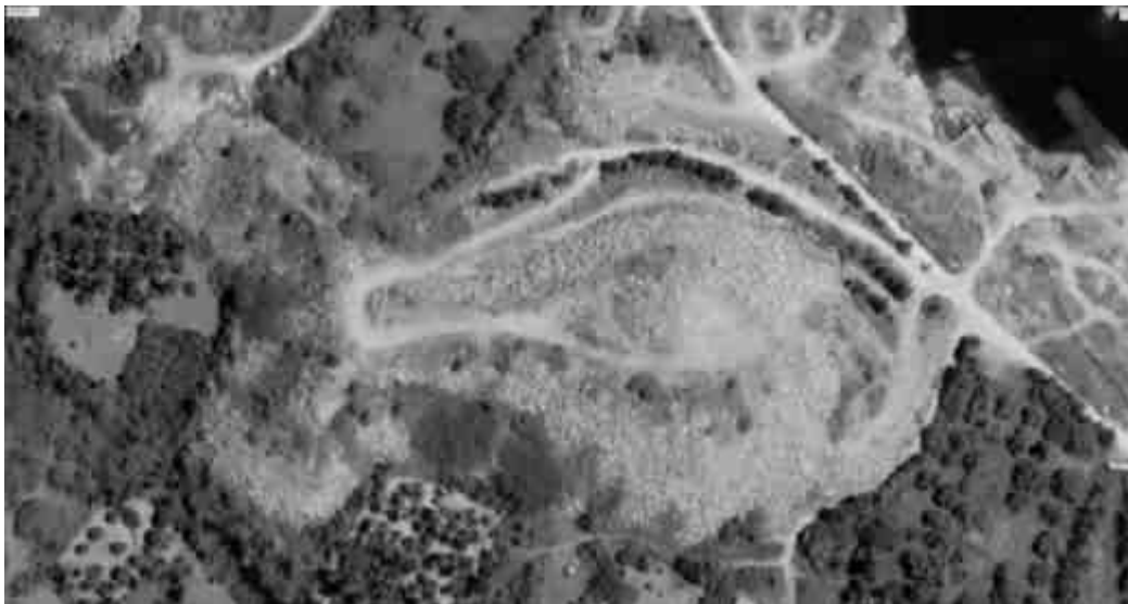
Fig No 13.3 Photos showing reject dump without garland drainage
