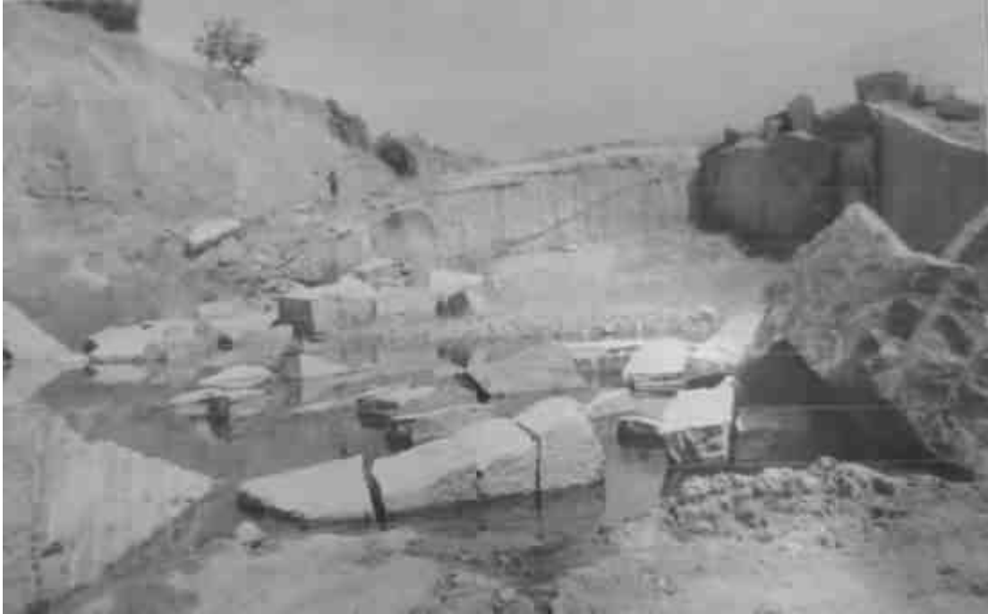
Fig. No. 2.5 General View of the existing lease area of M/s. Karunai Granites Private Limited.
