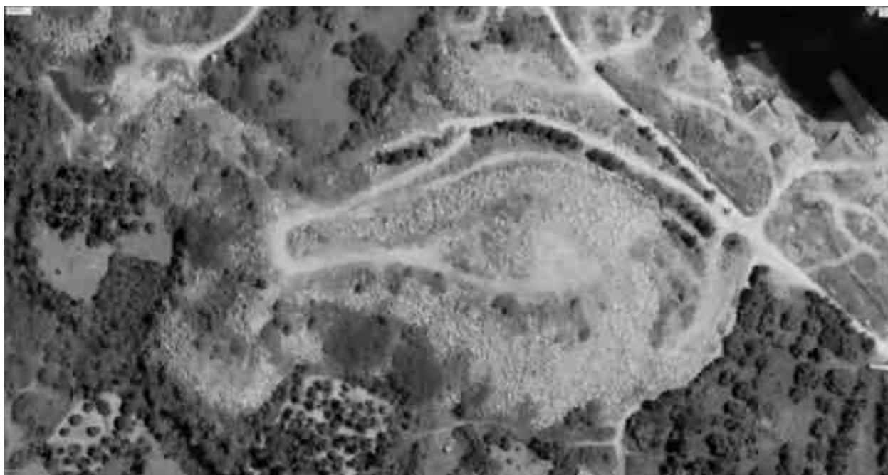
Fig No 13.1 Photos showing reject dump without garland drainage
