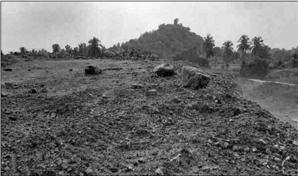
Figure 2.1 The overall view of the project site
