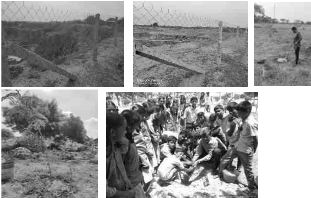
FIGURE 2.4: FENCING AND GREENBELT OF THE PROJECT SITE-P3
