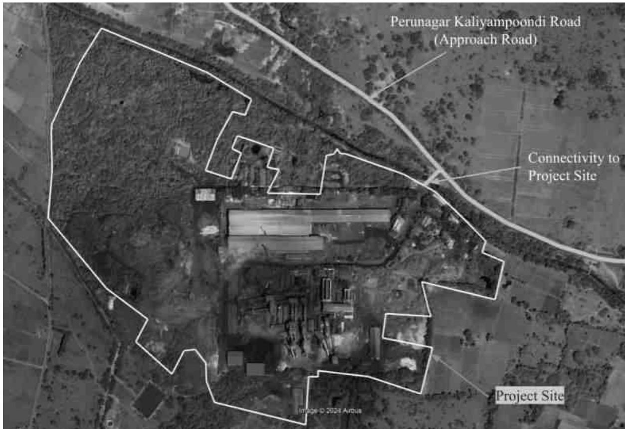
Figure 49. Approach Road to the Project Site
