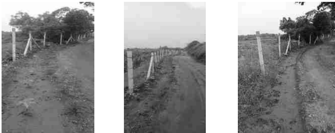
Fencing at Project site
