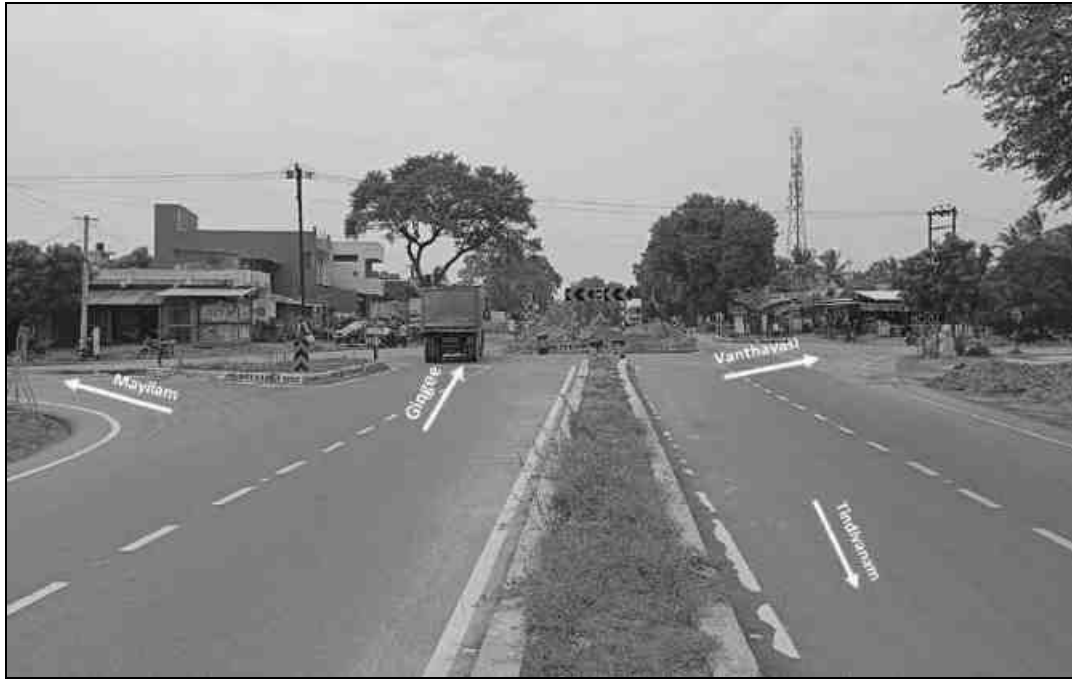
Figure 3-24 Photographs of Traffic monitoring location
