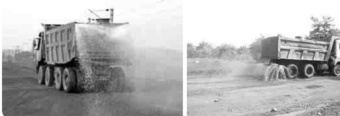
FIGURE 10.1: WATER SPRINKLING ON HAUL ROADS
