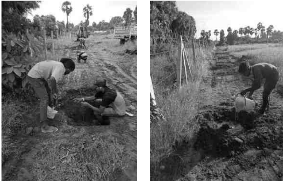
Fencing & Greenbelt at Project site
