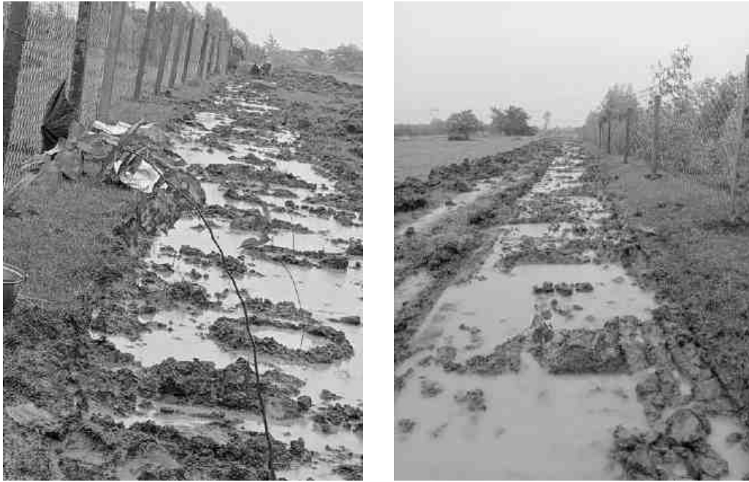
Fencing & Greenbelt at Project site
