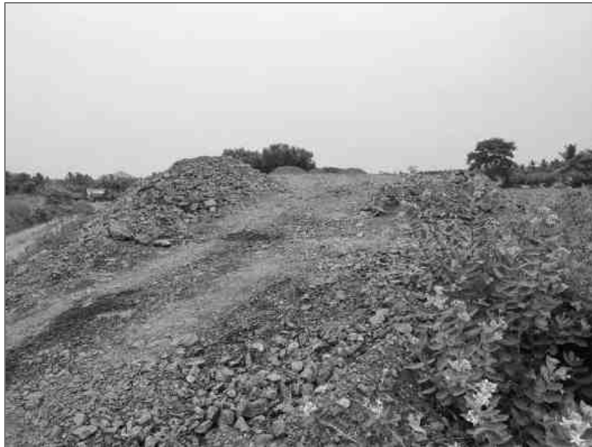
Crusher material stored temporarily in the project site
