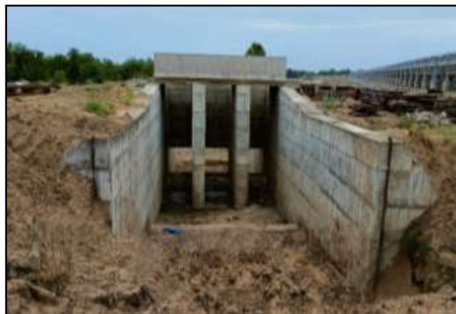
Fig No 1.2 Head sluice of south rajan channel
