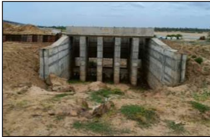
Fig No 1.1 Head sluice of north rajan channel
