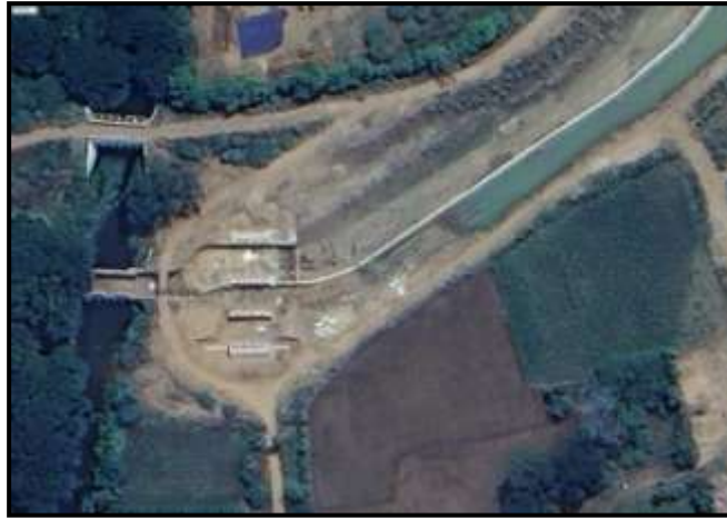
Fig No 1.3 Diversion of Narimudukku Drain into existing south rajan channel by constructing baffle wall at the centre of channel
